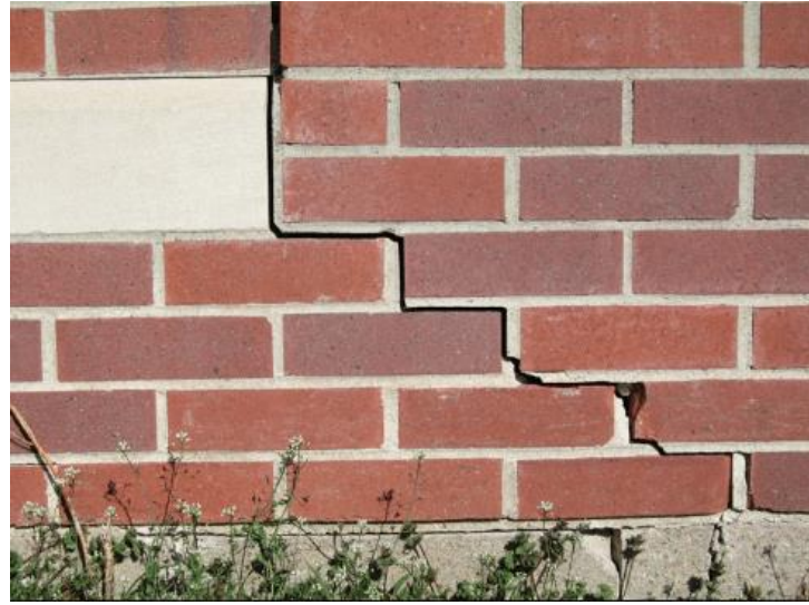
Exterior Cracks
