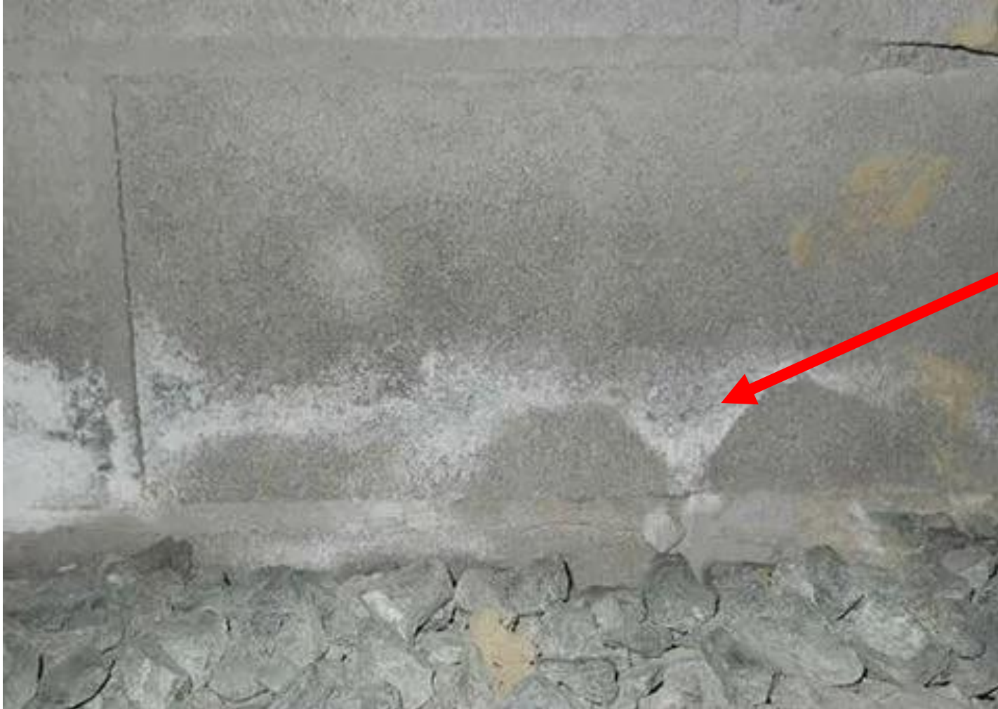
Efflorescence
