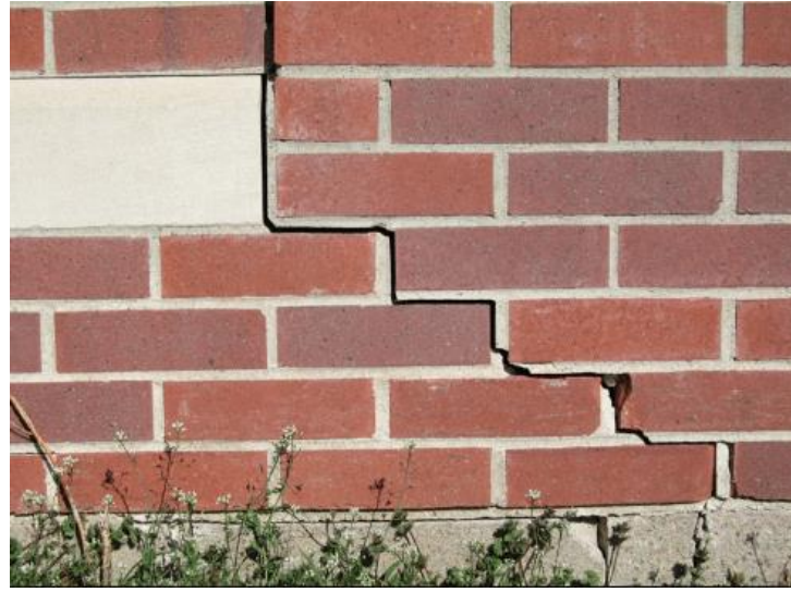
Exterior Cracks
