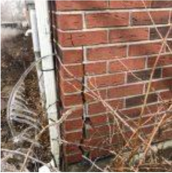
Exterior Cracks
