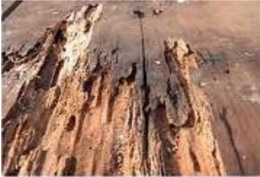
Termite Damage
