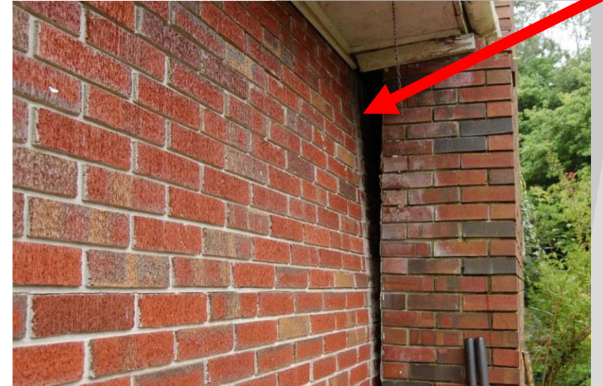
Chimney Separation
